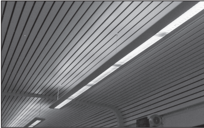
ceiling and lights in lower B hall
